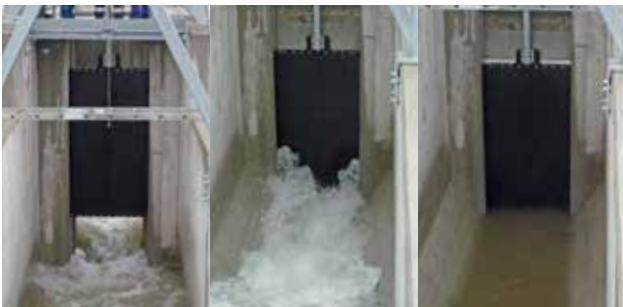
Electrically operated single-spindle penstock with handwheel for manual emergency operation and 4-side-sealing while closing the channel
