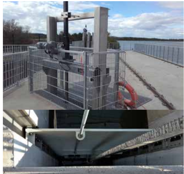
Penstock with electrically operated single rack drive and 3-side sealing
