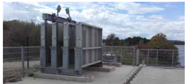
Penstock with electrically operated single rack drive and 3-side sealing
