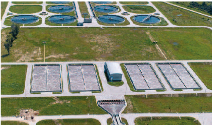
Central wastewater treatment plant of Zagreb, the capital of Croatia
