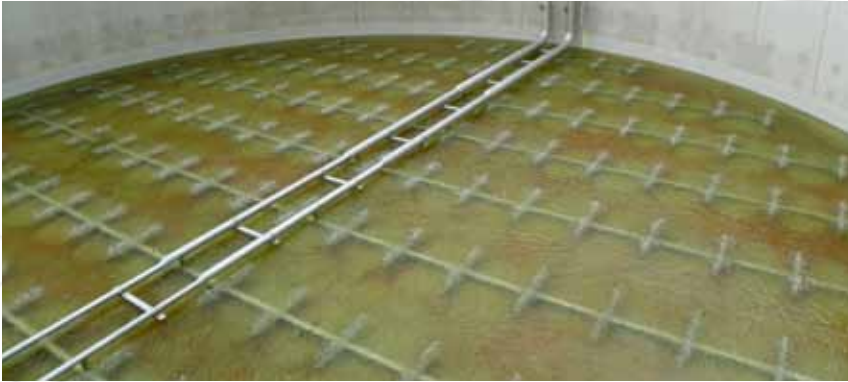
iCBA® aeration system during clearwater test in an industrial purification plant in France (dairy industry)
